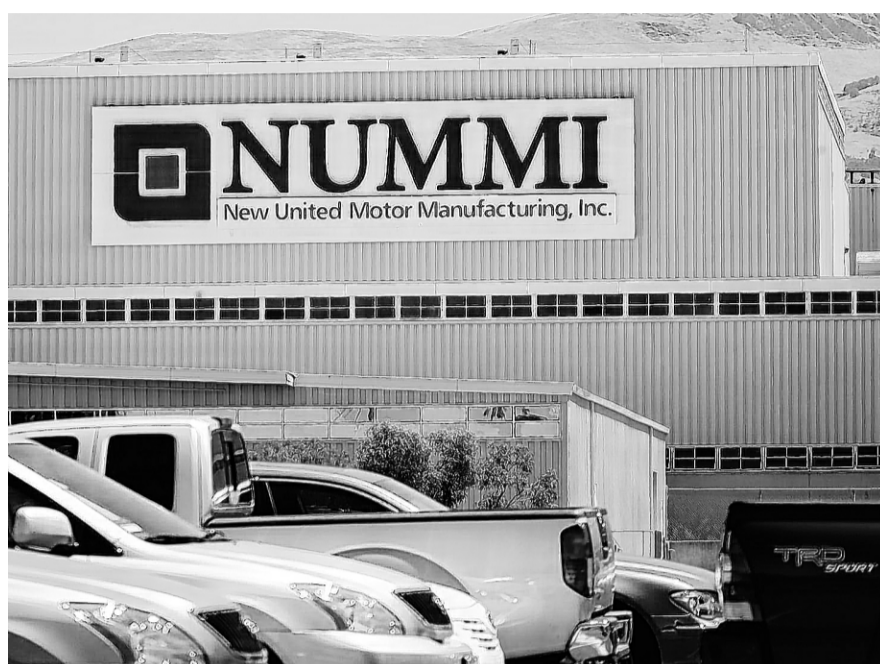
Toyota Motor Corp. has decided to liquidate its stake in the manufacturing plant in Fremont, Calif., that it jointly operated with General Motors, a Japanese news agency reported Thursday. PAUL SAKUMA / ASSOCIATED PRESS
